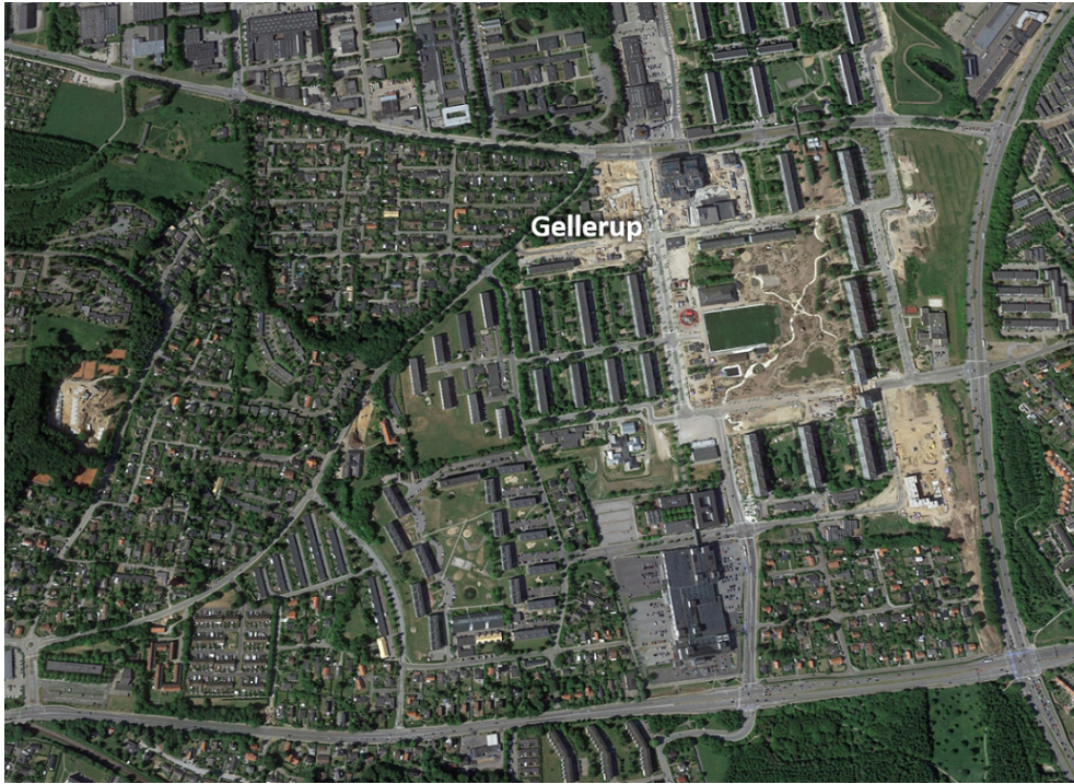
Figure 4.3. Aerial photo of Gellerup, one of the largest neighbourhoods that fulfils the ghetto criteria in Denmark. Empty spaces where demolition has taken place can be seen in the figure. In some of these spaces, construction has already been finalized. The student housing seen in figure 4.2 is one such example. Source: Google Earth
