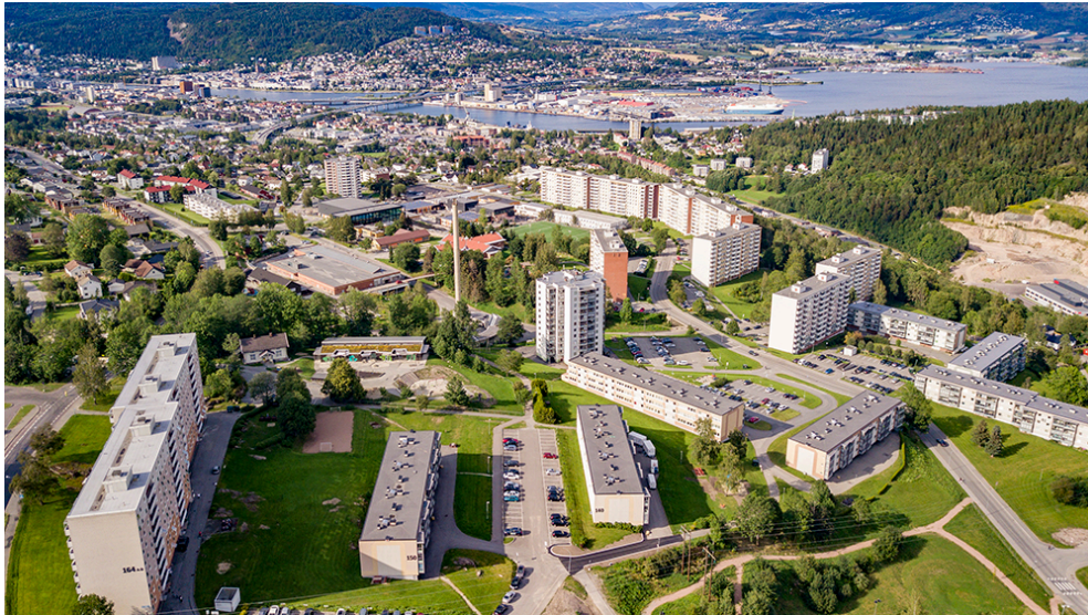
Figure 3.2. The variable local topography shows big differences in height. Source: Drammen Live24
