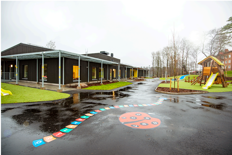
This picture shows a preschool in Borås designed with several measures to increase accessibility. The play area has no obstacles and the iron pillars on the front of the house provide enhanced visibility. There are parking space, elevator, a doorbell.
